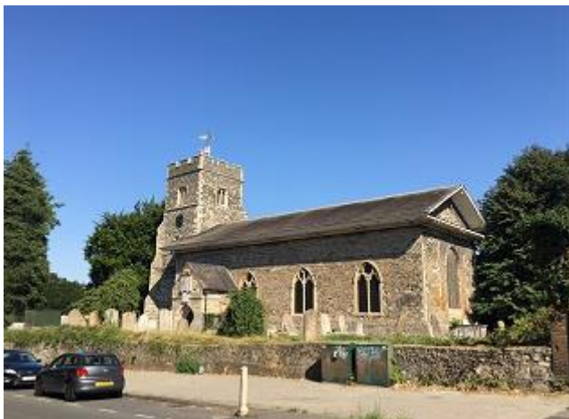
Flint section of the wall along East Milton Road
