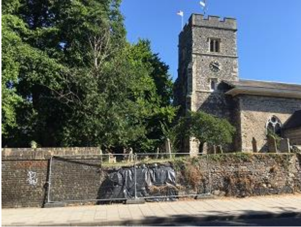
Close up of the collapsed and adjacent section of the flint wall to be rebuilt
